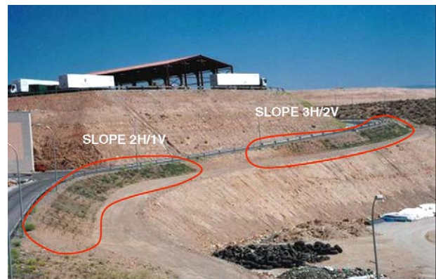
Fig. 2. General view of the experiment area.
